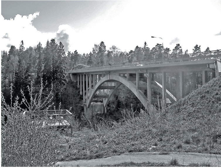
Bro i armerad betong.
